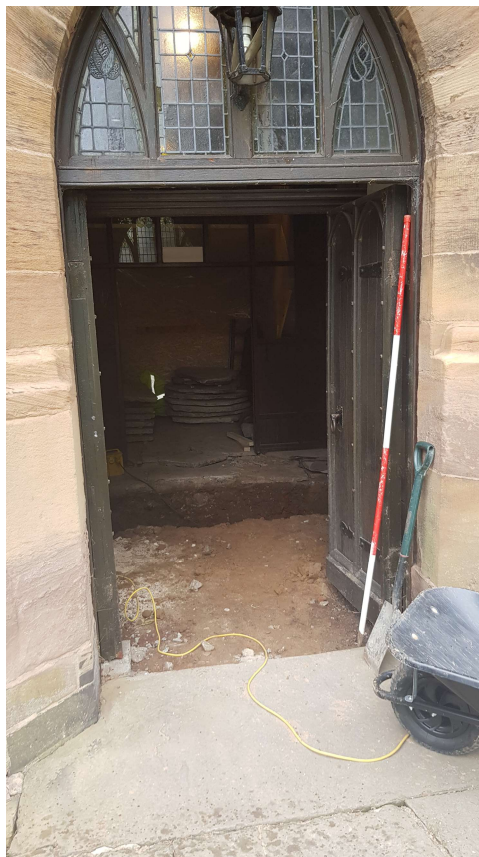
Plate 3 Tower entrance, facing east (scale 2x2m)
